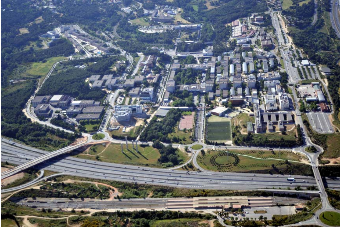
Fig. 5. The UAB is located in a natural setting of almost 200 hectares of green land and at the centre of a major communications network.
